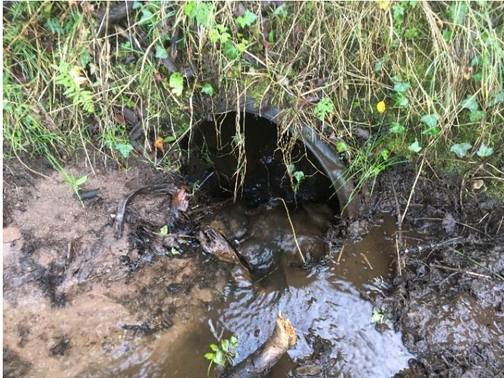
Watercrossing Structure W5
