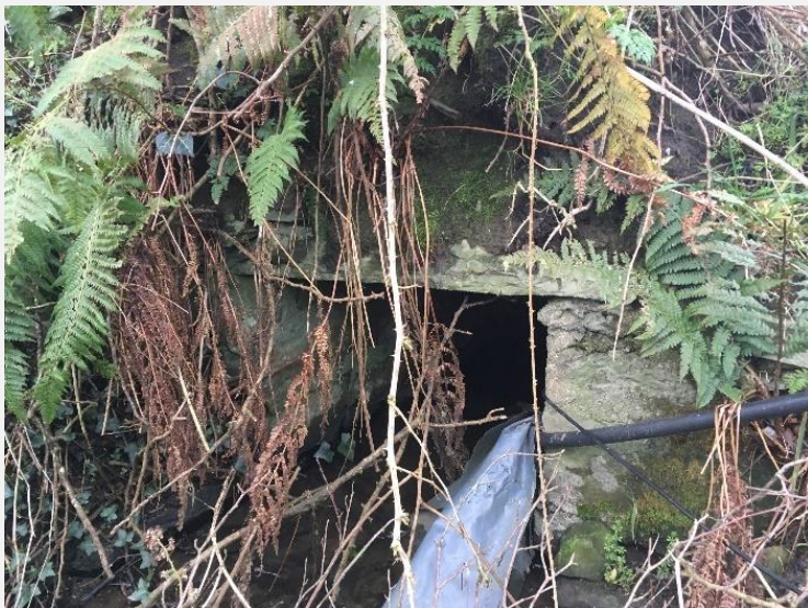
Watercrossing Structure W56
