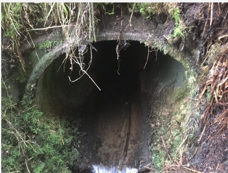
Watercrossing Structure W60
