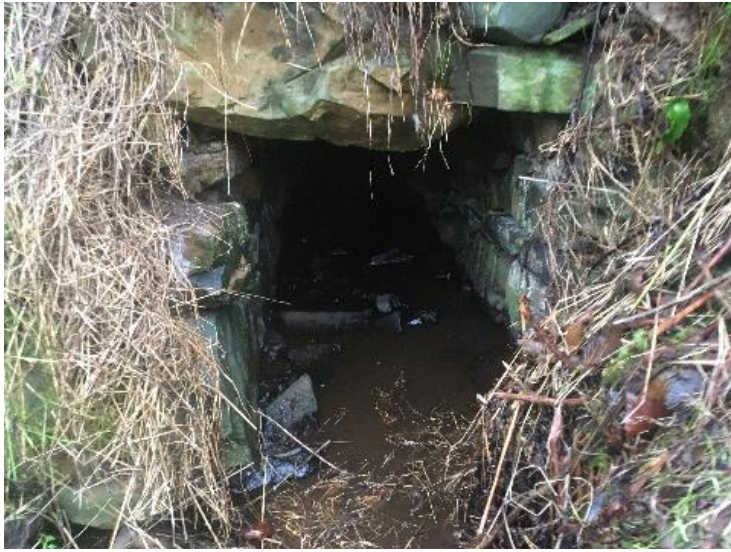
Watercrossing Structure W29
