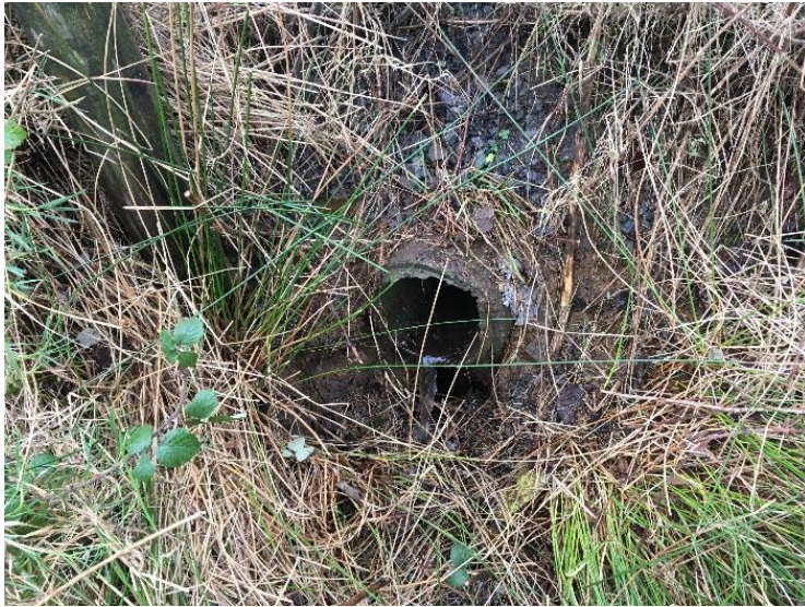
Watercrossing Structure W53
