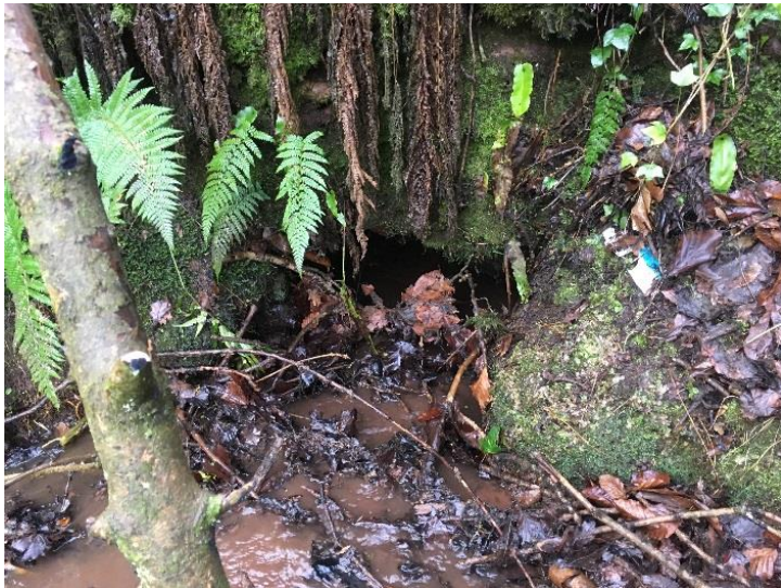
Watercrossing Structure W6
