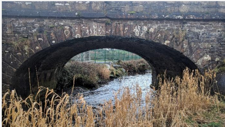
Watercrossing Structure W48
