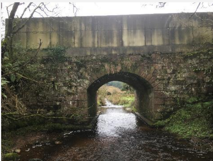
Watercrossing Structure W28
