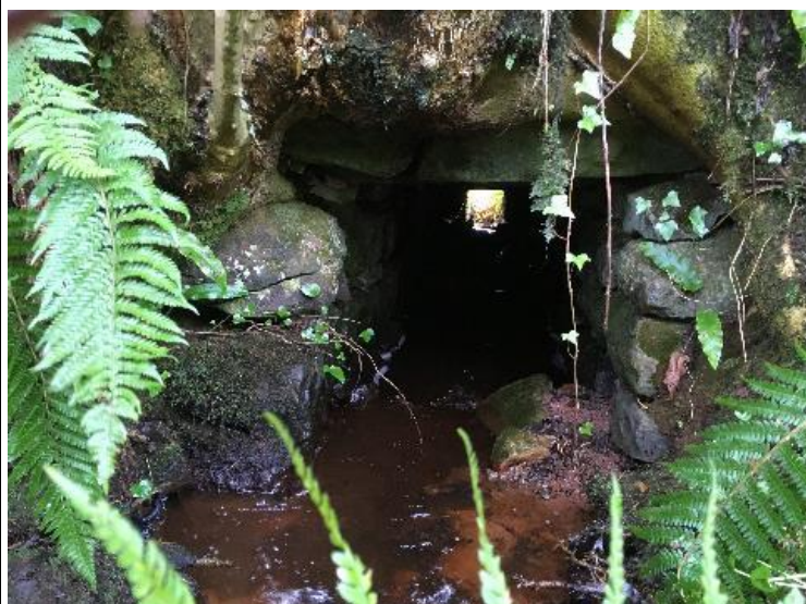
Watercrossing Structure W10
