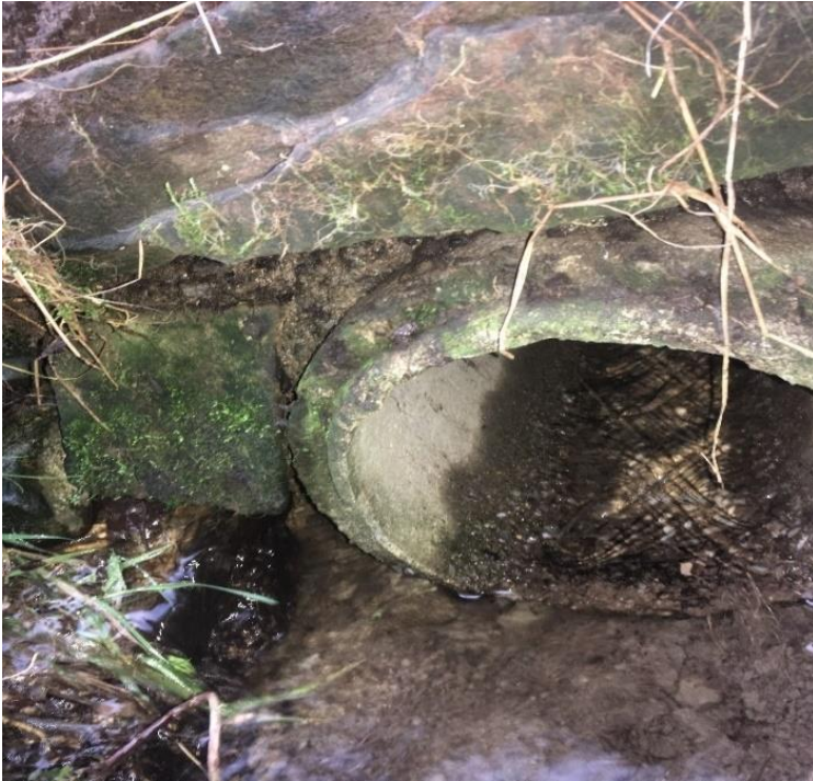
Watercrossing Structure W61
