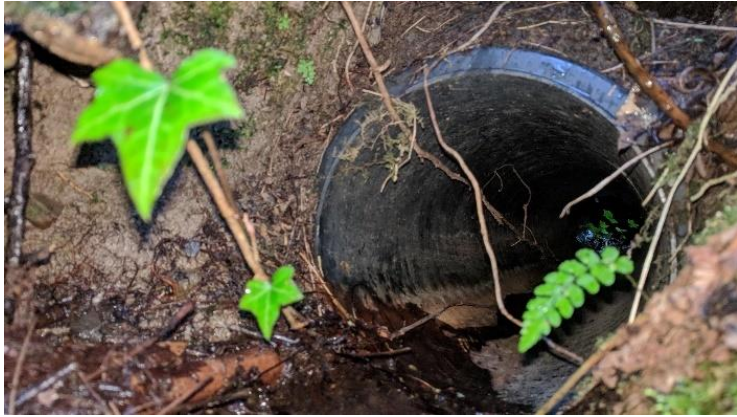
Watercrossing Structure W49
