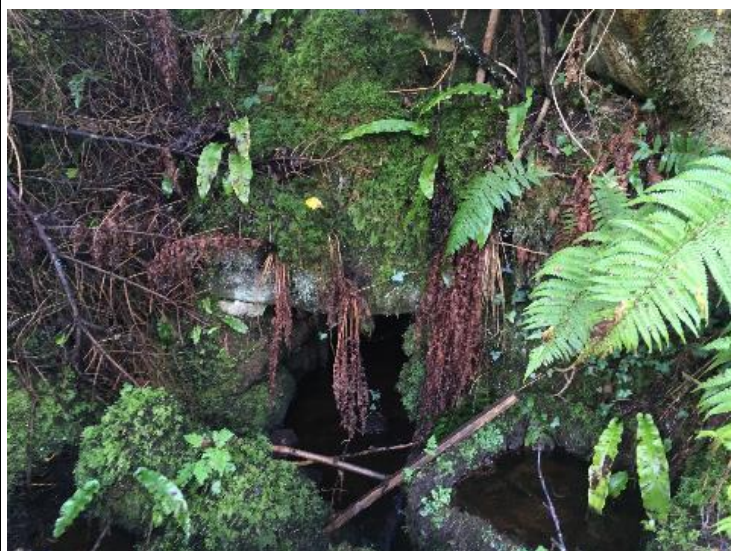
Watercrossing Structure W8
