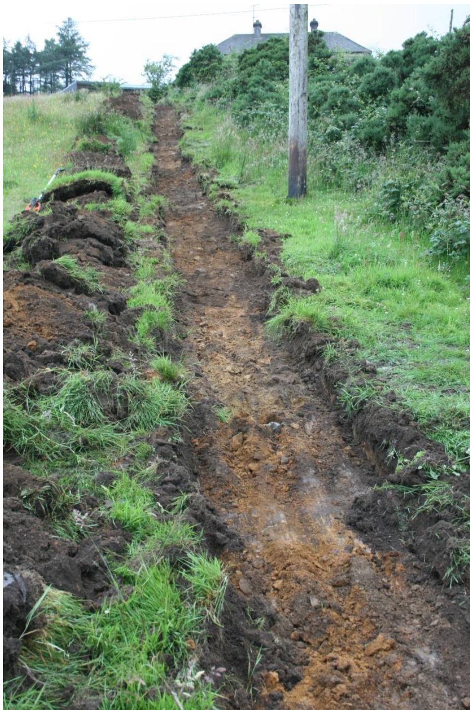
Figure 4: Trench 1 from the southeast
