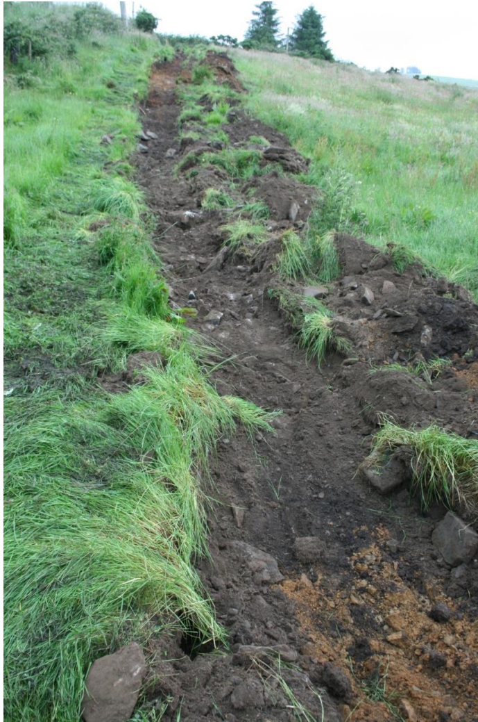
Figure 7: Trench 2 from the southwest. Spread of mixed demolition rubble visible in the foreground
