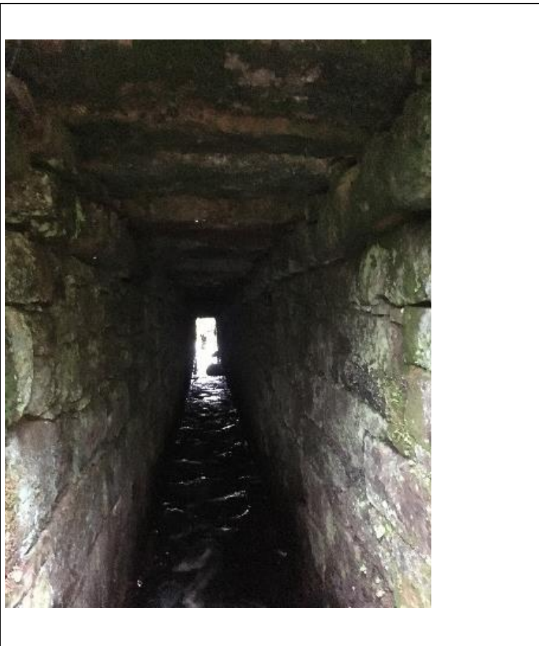
Watercrossing Structure W13
