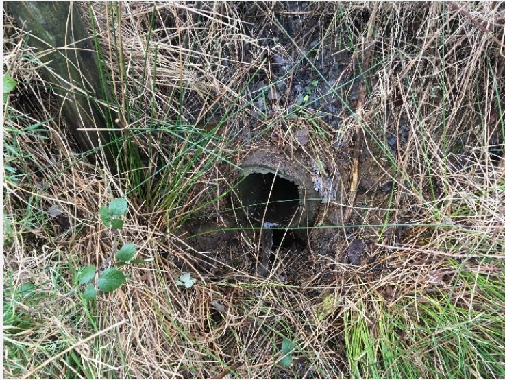
Watercrossing Structure W51
