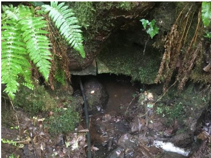
Watercrossing Structure W26
