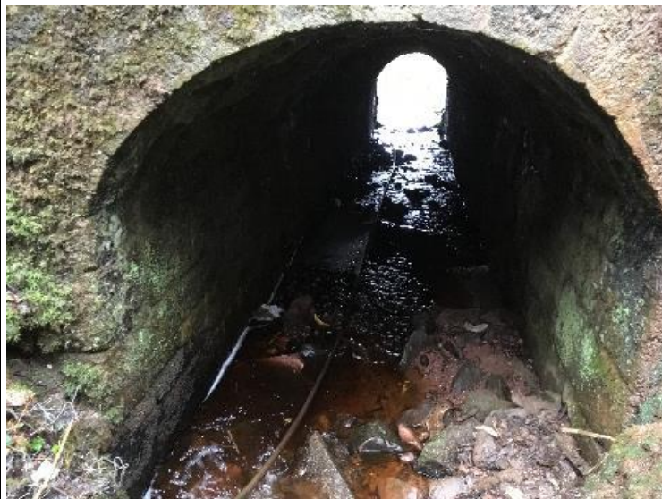
Watercrossing Structure W17
