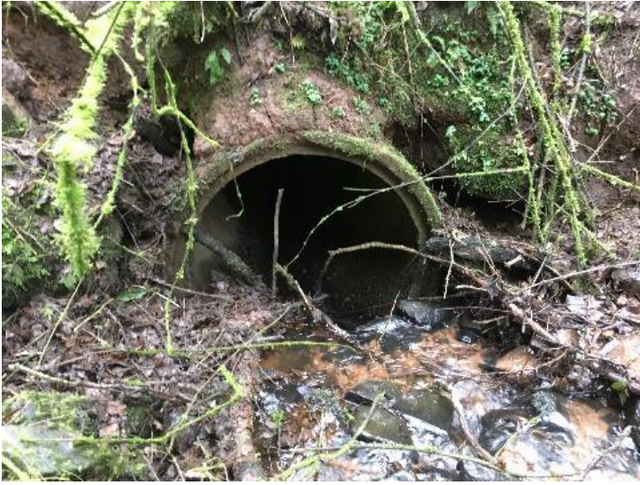
Watercrossing Structure W19
