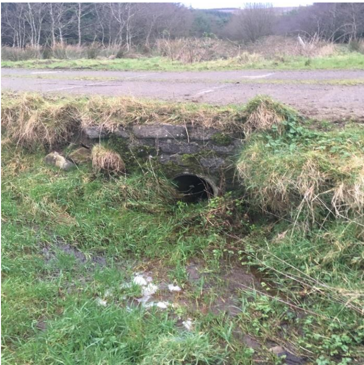
Watercrossing Structure W62
