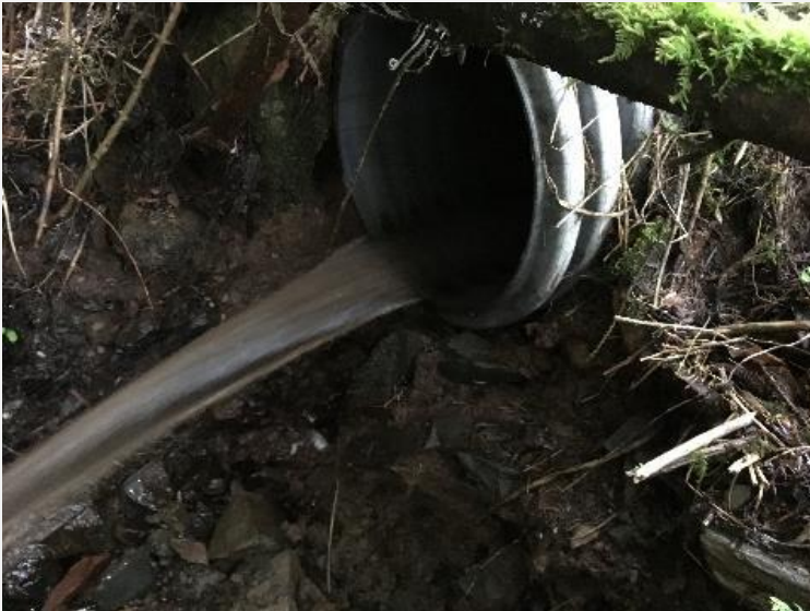
Watercrossing Structure W20
