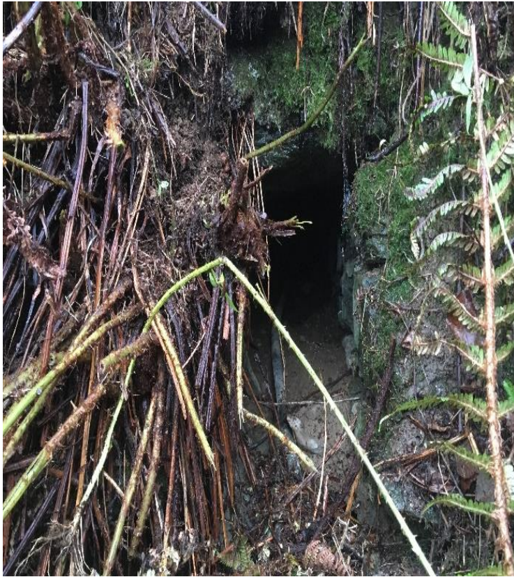
Watercrossing Structure W57
