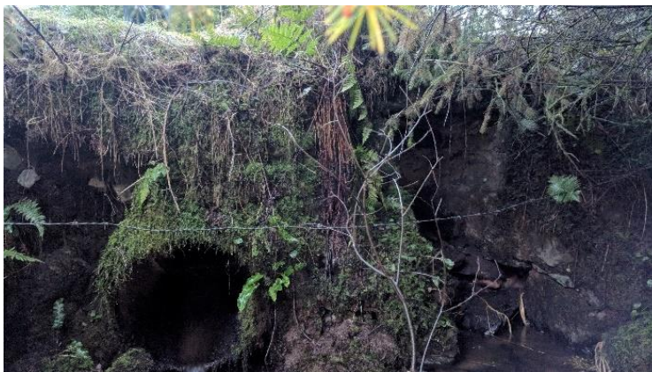
Watercrossing Structure W54
