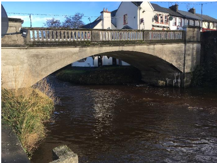
UWF Grid Connection Bridges / Culverts
