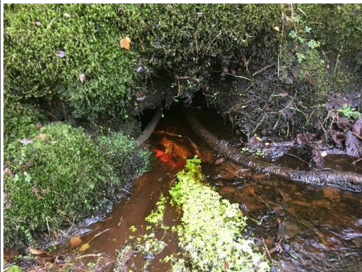
Watercrossing Structure W14
