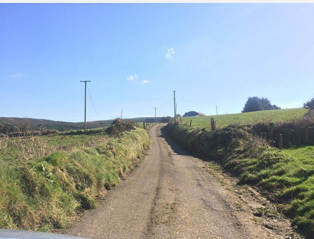
UWF Related Works Internal Windfarm Cable Public Road Crossings RW4 & RW5
