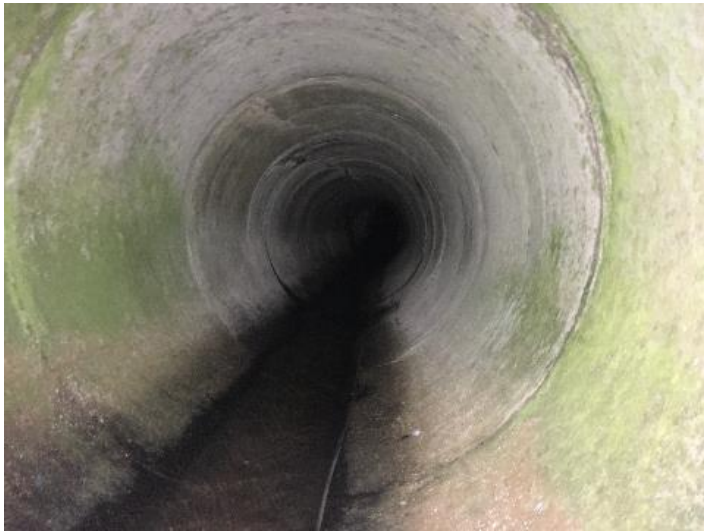
Watercrossing Structure W21
