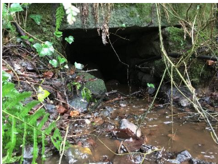
Watercrossing Structure W12
