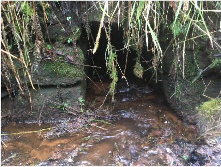
Watercrossing Structure W27
