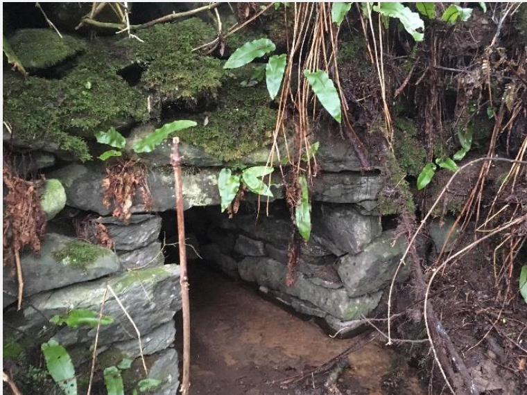
Watercrossing Structure W59
