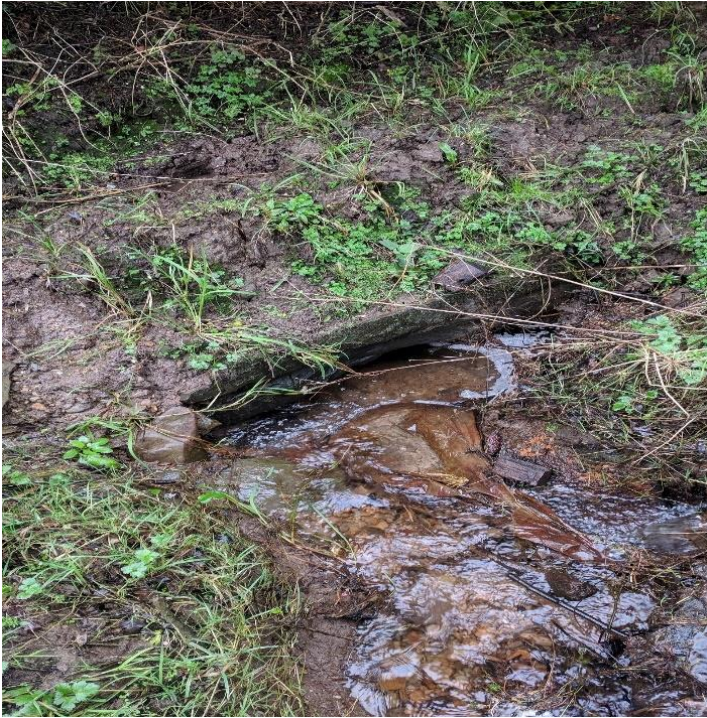
Watercrossing Structure W37
