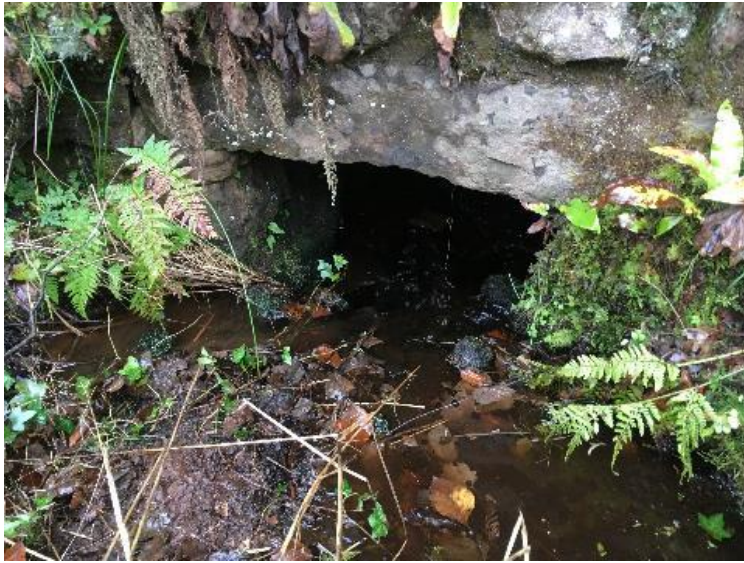
Watercrossing Structure W15
