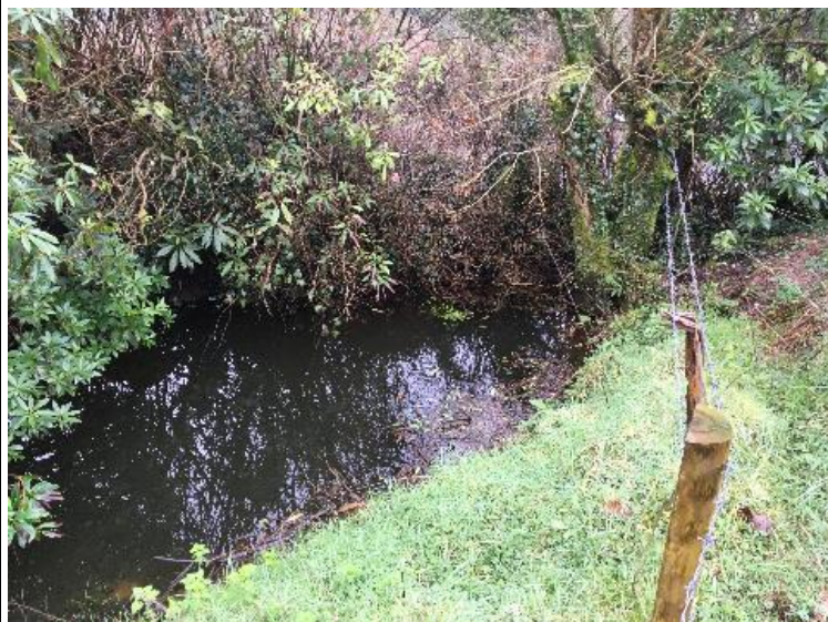
Watercrossing Structure W11
