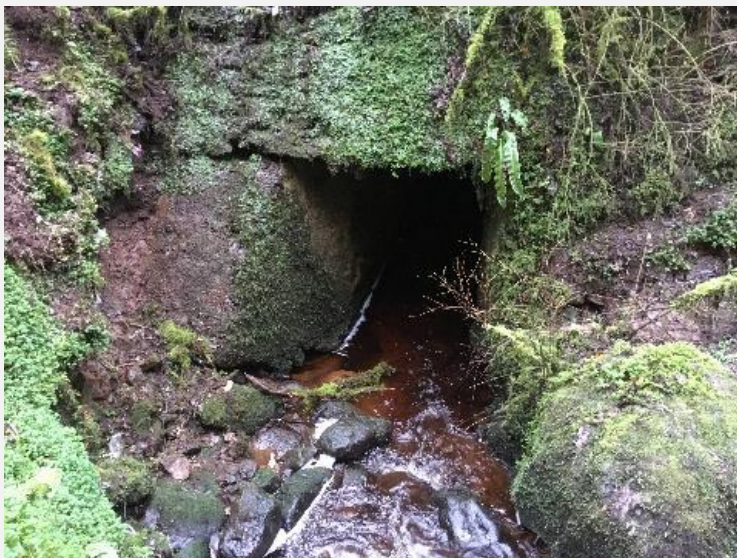
Watercrossing Structure W24
