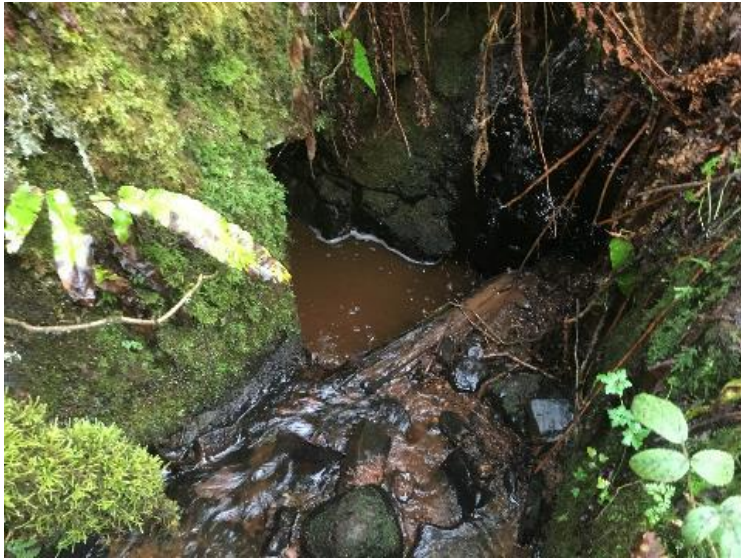
Watercrossing Structure W25
