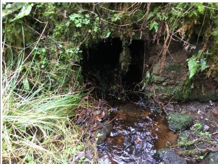
Watercrossing Structure W9
