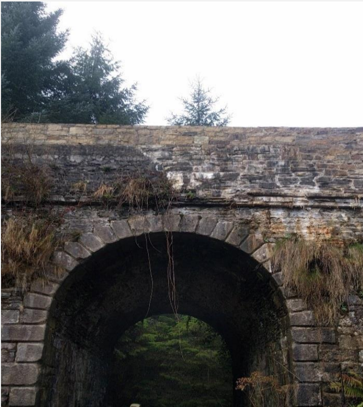
Watercrossing Structure W44
