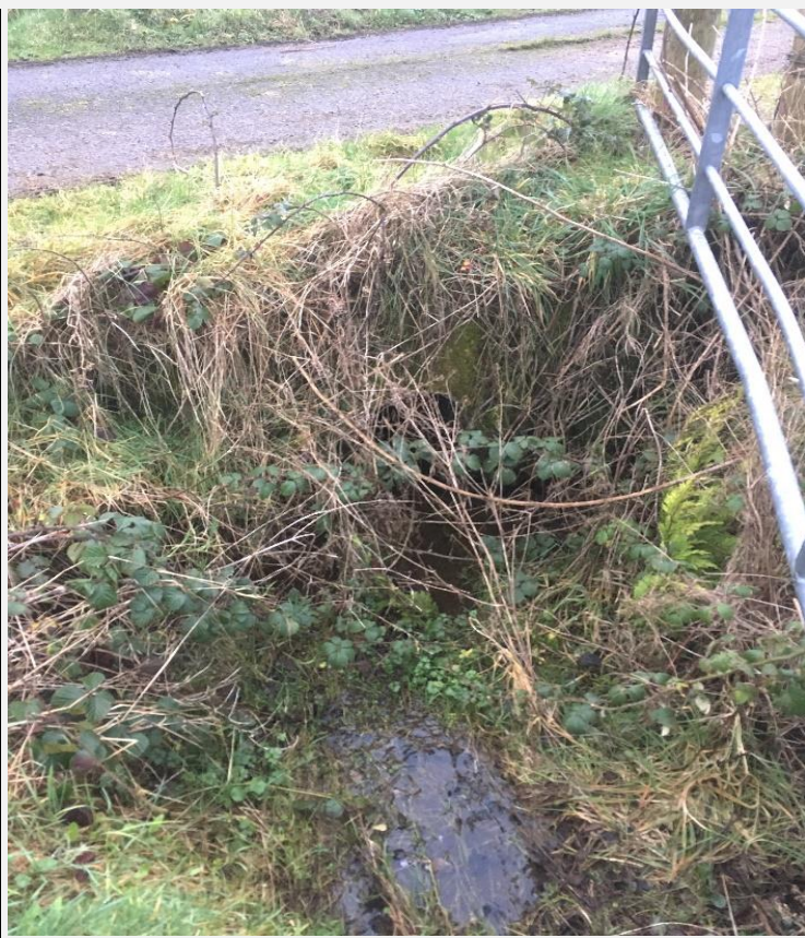
Watercrossing Structure W63
