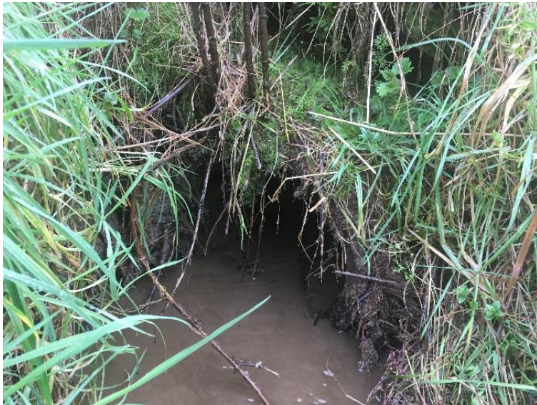
Watercrossing Structure W58
