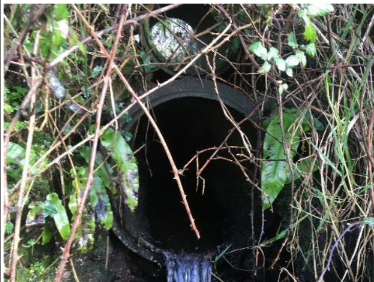
Watercrossing Structure W7
