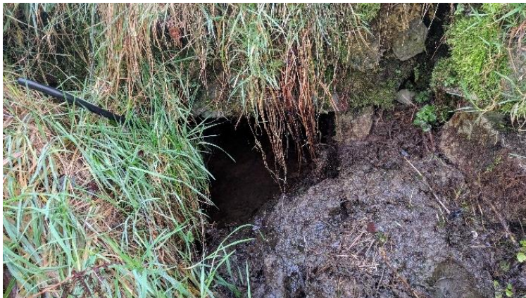
Watercrossing Structure W50
