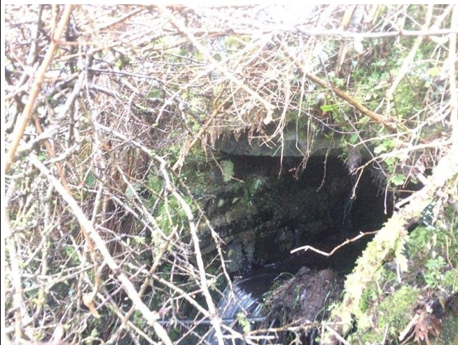
UWF Related Works Haul Route Works Bridge/Culvert Crossings WW32
